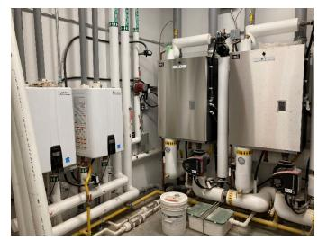
New high efficiency, on-demand hot water heating (L) and boilers (R) at wəkwanəs tə syaqwəm Elementary School
