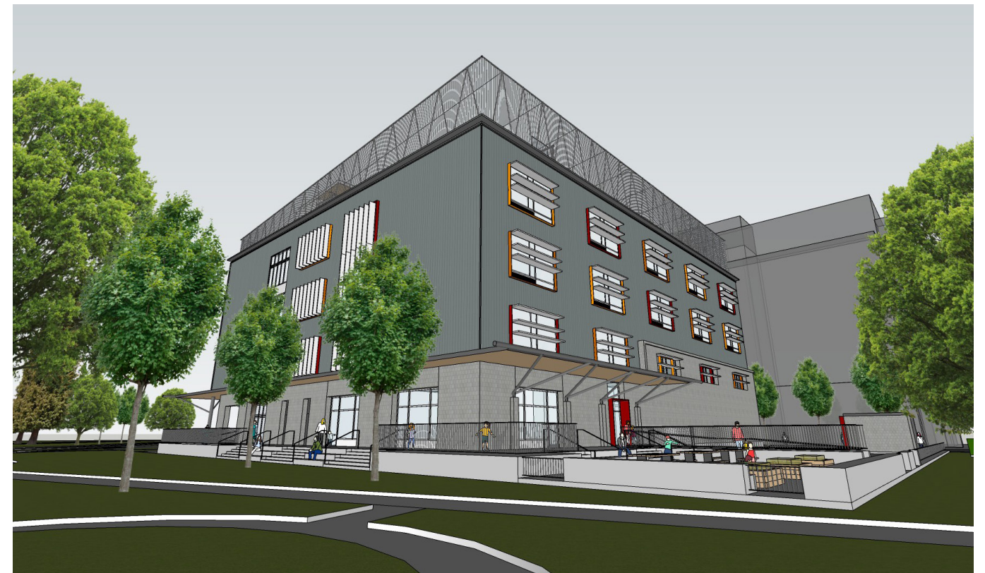
View from south-west showing the light play area guards and netting
