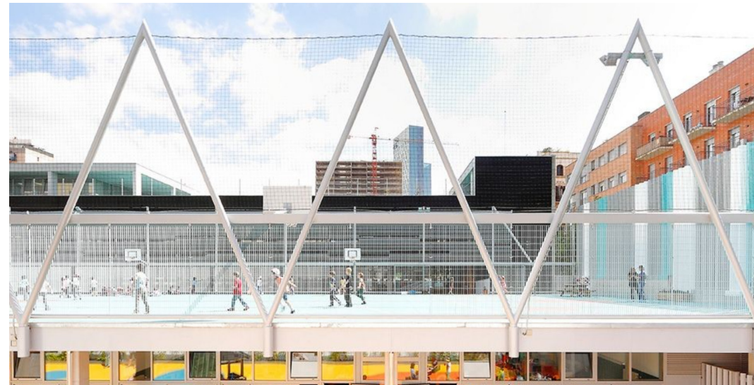
Roof-top steel braces and fencing
