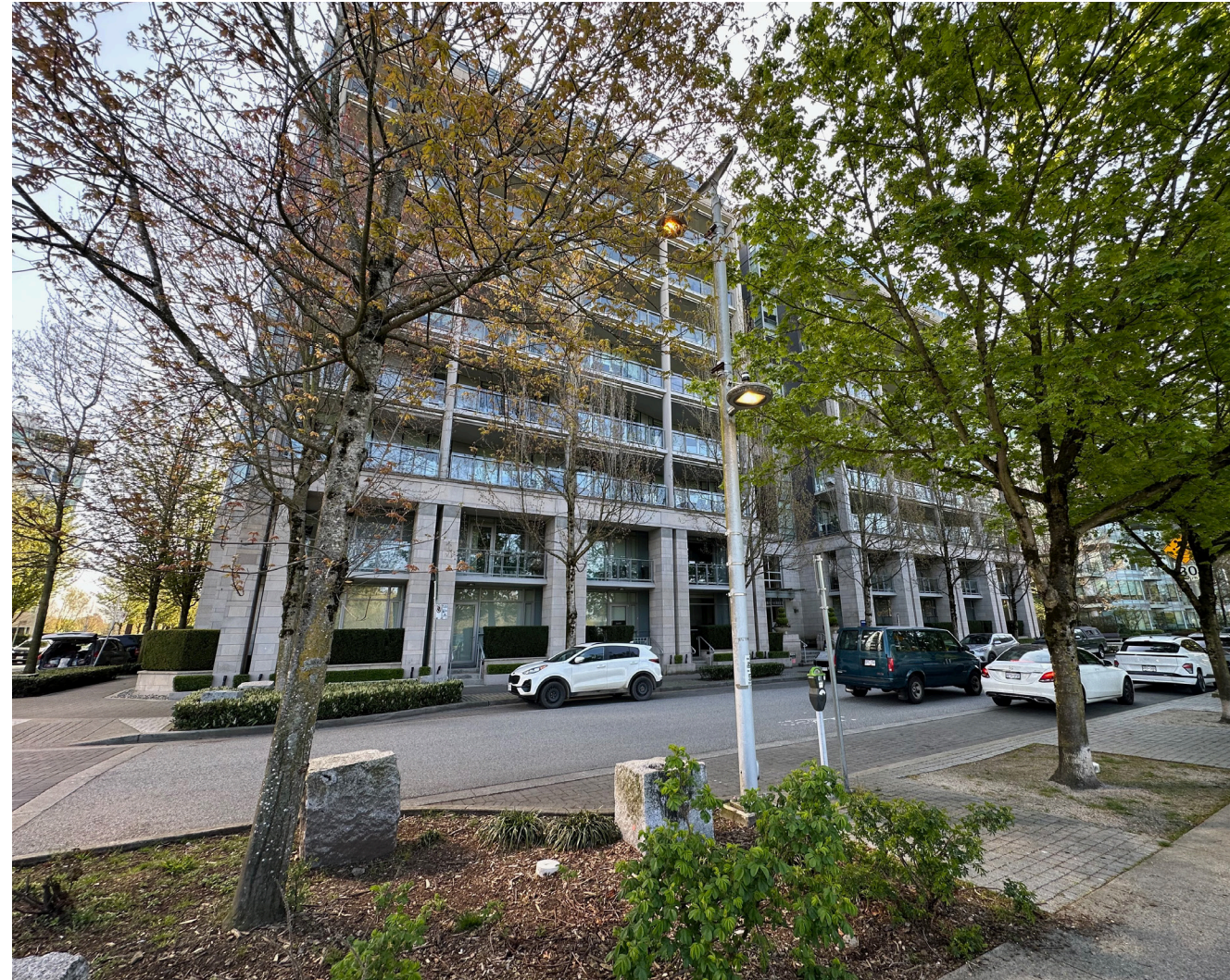
Neighbouring building across from Columbia Street: The streetwall on Columbia has a 2 storey datum line of stone materials. This material and height is reflected on the school facade facing Columbia Street.
