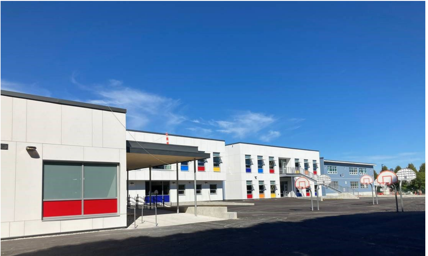
Upgraded seismically safe school - Weir Elementary
