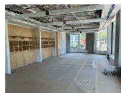
Photos of the new school currently under construction
