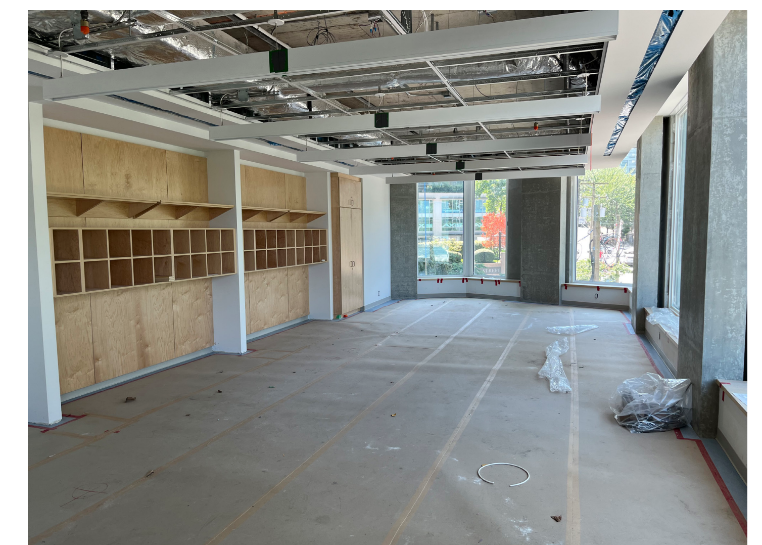
Photos of the new school currently under construction
