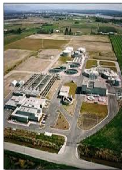
Lulu Island WWTP
