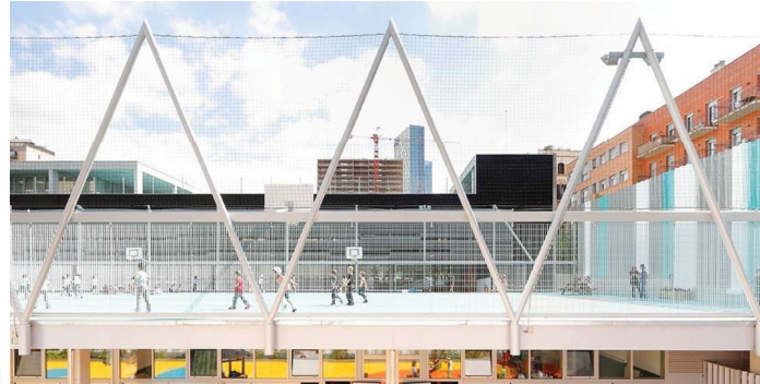
Roof-top steel braces and fencing
