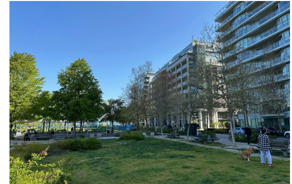
Residential buildings along Columbia Street
