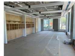
Photos of the new school currently under construction
