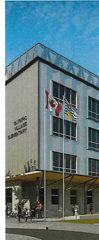
View from the north east, showing the front facade.
