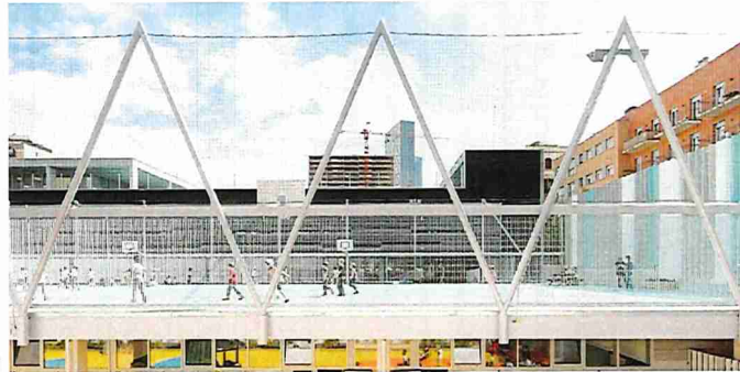
Roof-top steel braces and fencing
